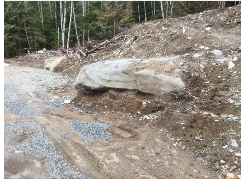
Remove large boulder to improve left approach alignment
