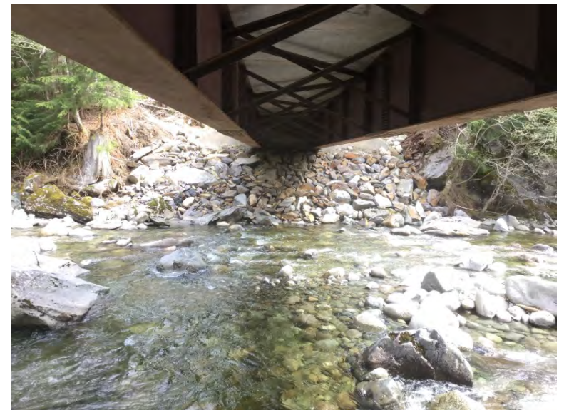
Left Bank Abutment when facing downstream
