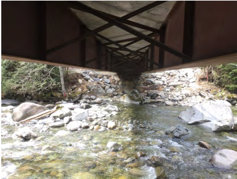
Right Bank Abutment when facing downstream
